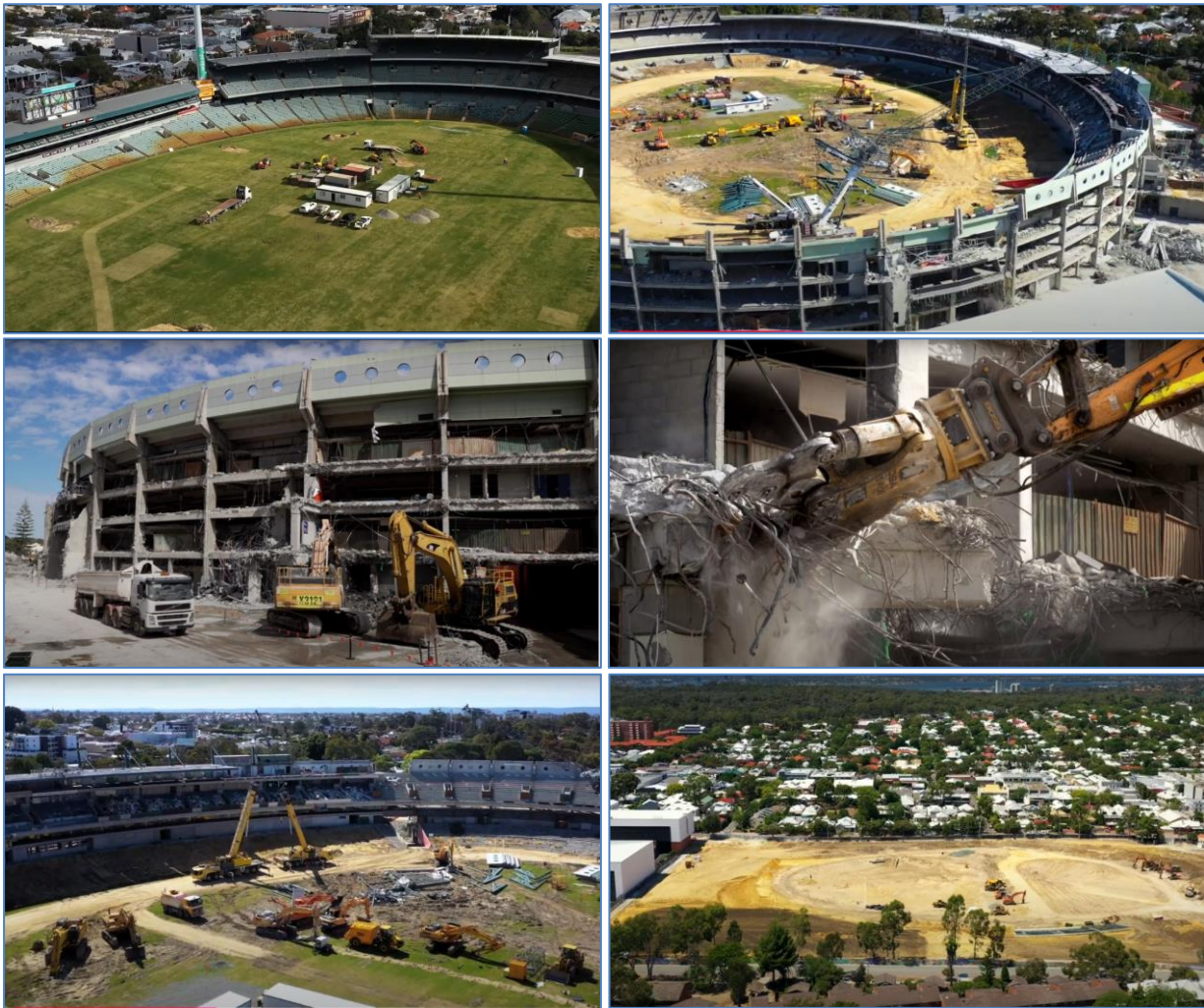
Figure 2. Overview of demolition activities in Subiaco Oval stadium project Source: Development WA (2021)
