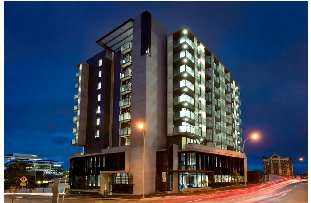
5 Green Square Close – supplied by Brisbane Housing Company
