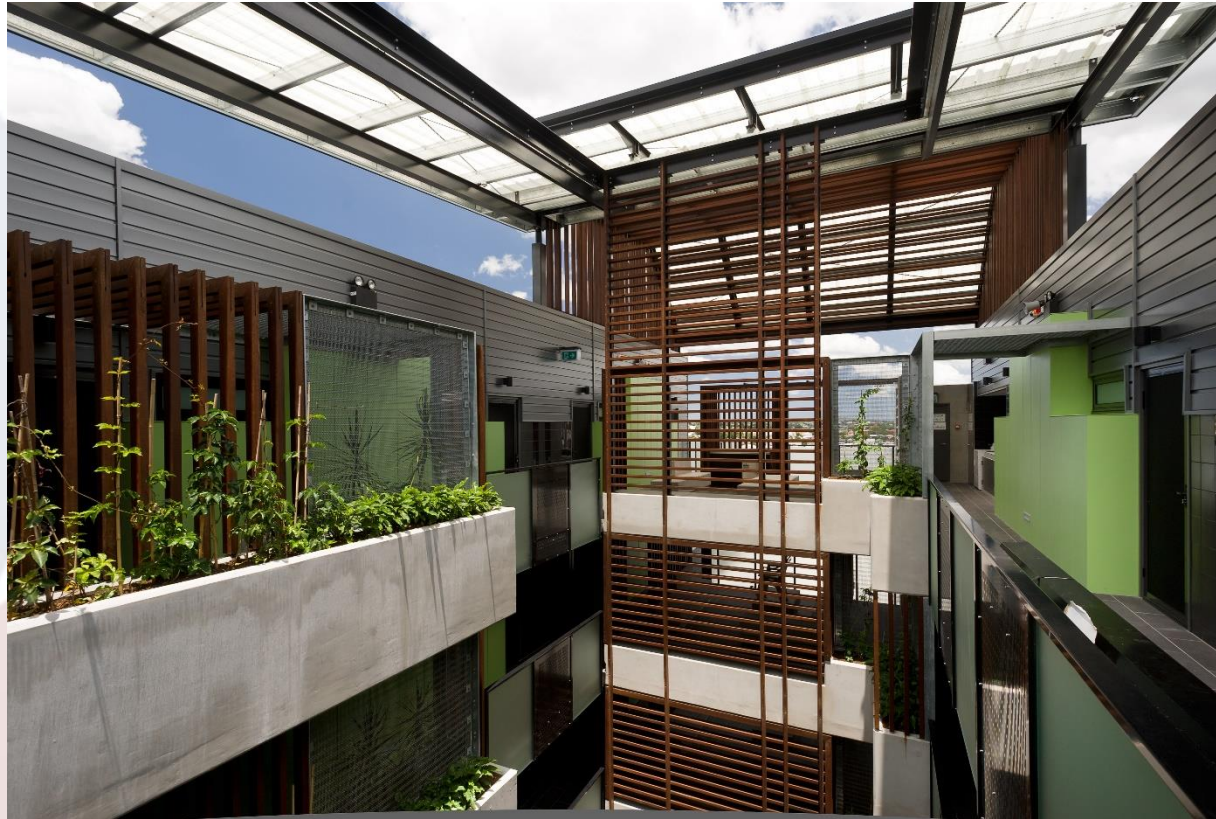
5 Green Square Close – supplied by Brisbane Housing Company
