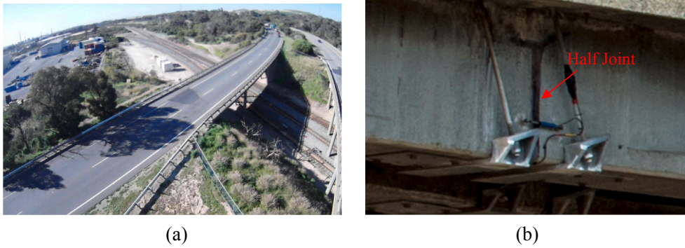
Fig. 15. An operational highway bridge: (a) Bird view of the bridge; (b) The reinforced half joints.
