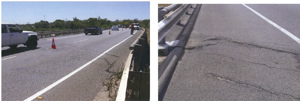
Fig. 22. The damaged surface of the bridge deck.
