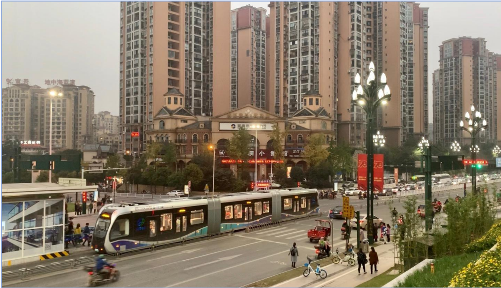
Figure 9: Trackless tram in operation in Yibin, Sichuan Province, China
