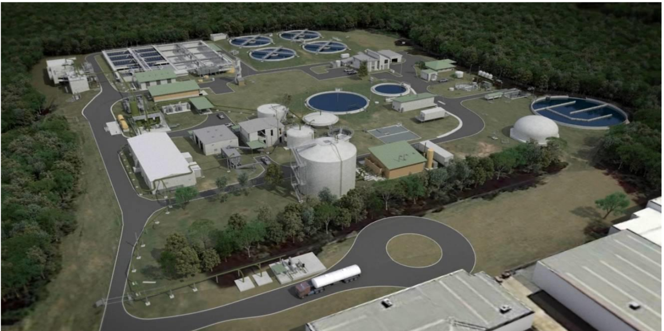
Figure 4: Kawana Sewage Treatment Plant (Kent and Smith, 2019)
