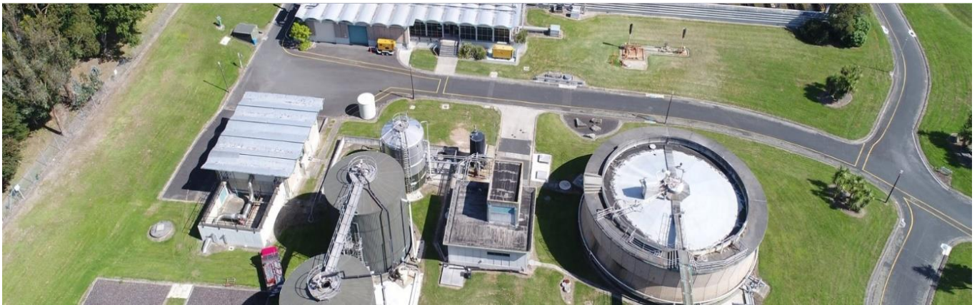
Figure 1: Hamilton City Council Wastewater Treatment Plant (Hamilton City Council, 2020)
