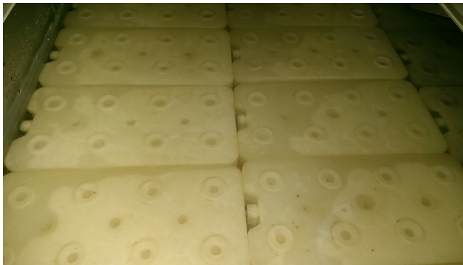
Fig. 4. FlatICE PCM blocks inside the PCM tank.
