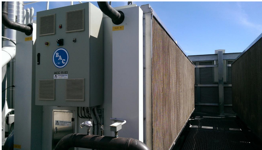
Fig. 6. Adiabatic cooler of the CCW system.
