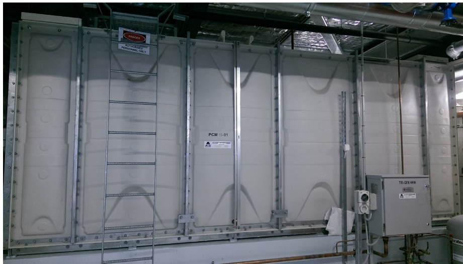
Fig. 2. Phase change materials tank in the case study building.
