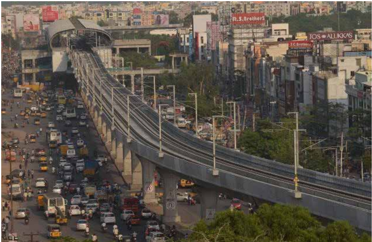
Hyderabad Metro in India. Source: The Hindu Business Line
