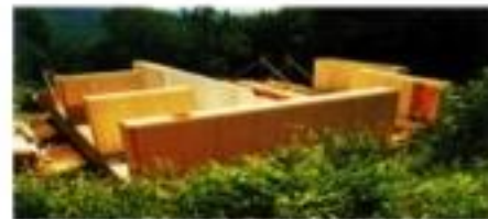
Figure 2.1.1.2 Furniture House by Shigeru Ban: Ban used panelized structures for the interior structural skeleton of the building (McQuaid 2003, 167).
