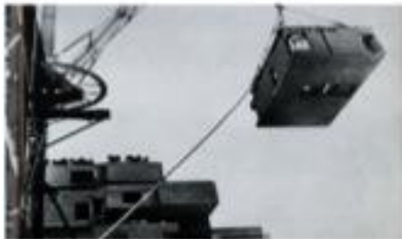
Figure 2.1.1.1 Habitat 67 by Mosche Safdie: Habitat is an assembly of prefabricated concrete modules (Safdie 1970, 23).
