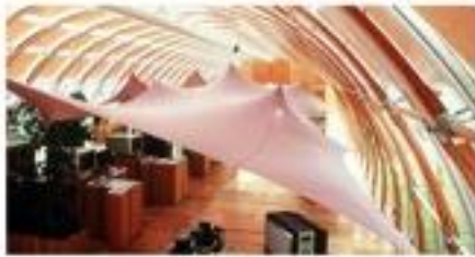
Figure 2.1.1.3 IBM Traveling Pavilion by Renzo Piano: This was a moving exhibition that was broken down into a series of prefabricated components that were designed with demountability and reassembly in mind (Dini 1984, 79).
