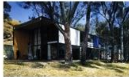
Figure 2.1.1.4 Eames House by Charles and Ray Eames: The Eames house was famously designed to be built from "off-the-shelf" standardized materials as much as possible (Smith 2007, 23).
