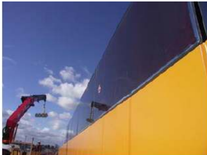
Figure 2: Solar panels on noise walls, (Johnston 2007)
