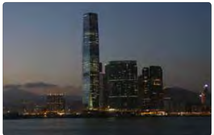
(Above): Hong Kong skyline with ICC building. Copyright Baycrest; (Top): Access to International Commerce Centre.
