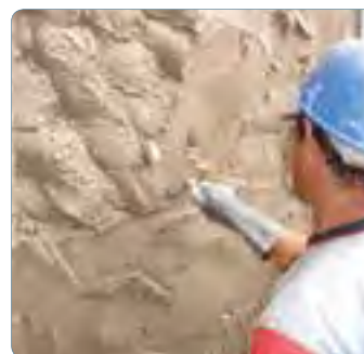
(Above): Facade surface conditioning to receive the mortar coating; (Left): Manual application of mortar coating.
