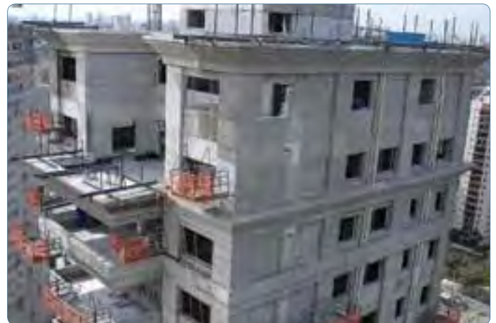
(Above): Facade surface conditioning to receive the mortar coating; (Left): Manual application of mortar coating.
