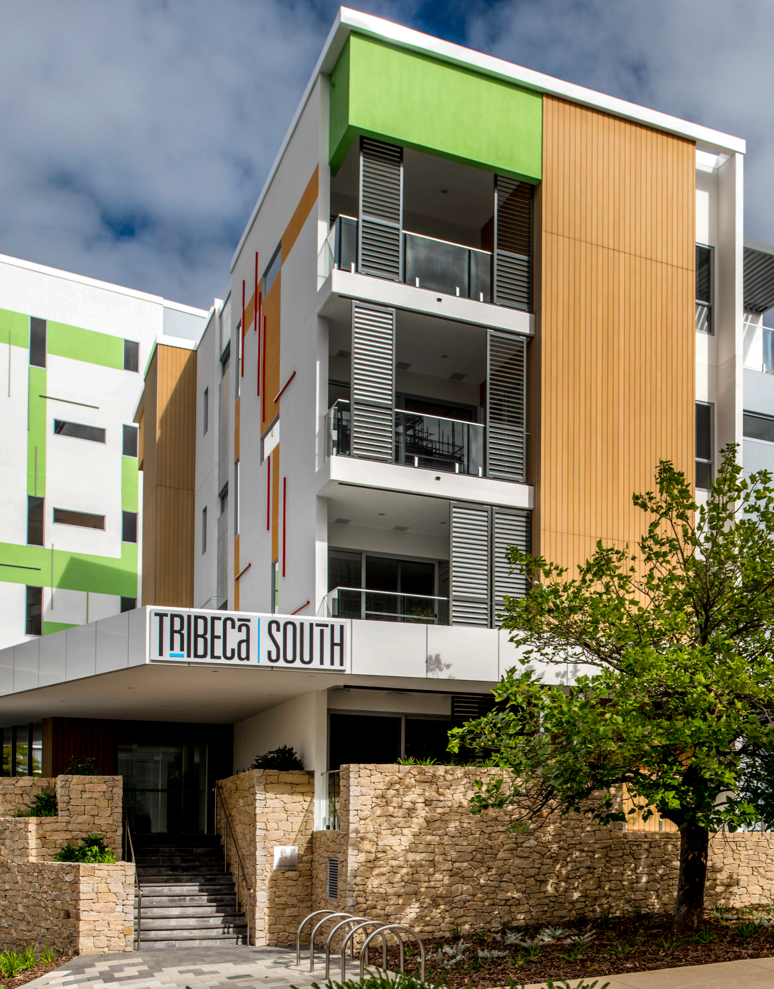
Tribeca South Apartments, WA (Source: BGC Construction)
