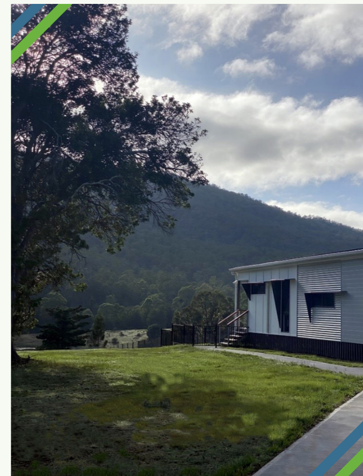
Modular prefabricated home delivered in Queensland in 2022/2023 (location confidential) Luke Rowlinson – Creating Positive Futures & Rowlinson Architects (Source: Shared with permission of the housing operator and lead contractor)
