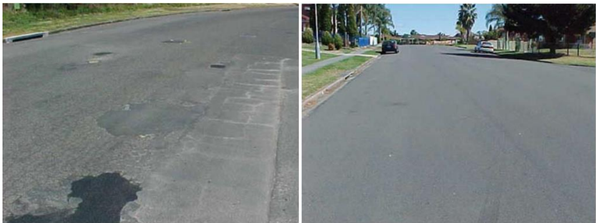
Figure 7. Road conditions before and 7 years after reclimation with crushed concrete Source: IPWEA NSW (2010) 14
