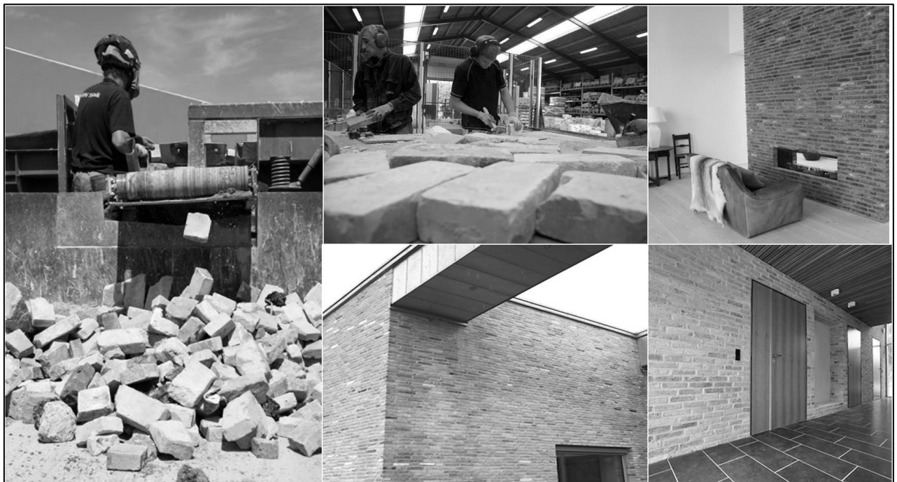
Figure 10. EBRICKS project operation and some examples of building with re-used (cleaned) bricks
