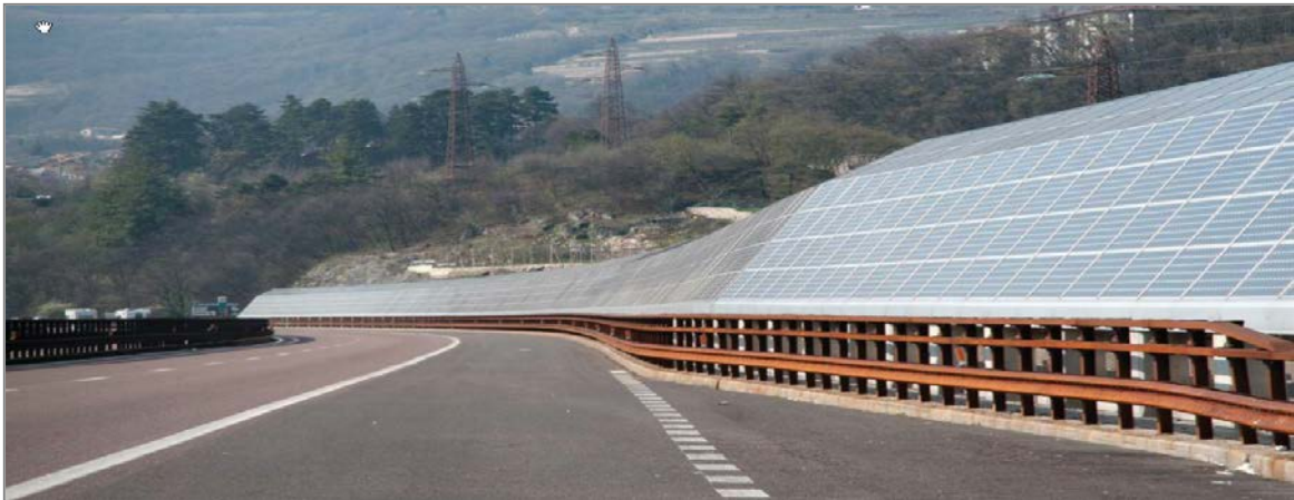
Figure 2: A photovoltaic noise barrier installed along the A22 Autostrada, Italy.
