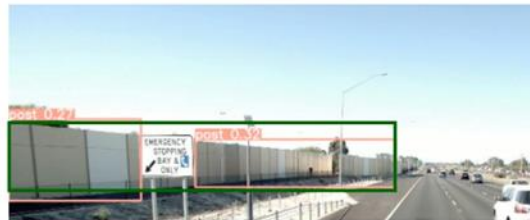
Walls blocked by signs
