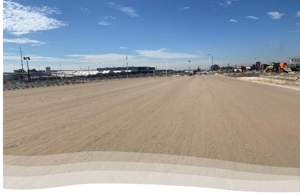
Use of CRC in a roadwork during mixture and compaction (left) and after trimming and sweeping (right)
