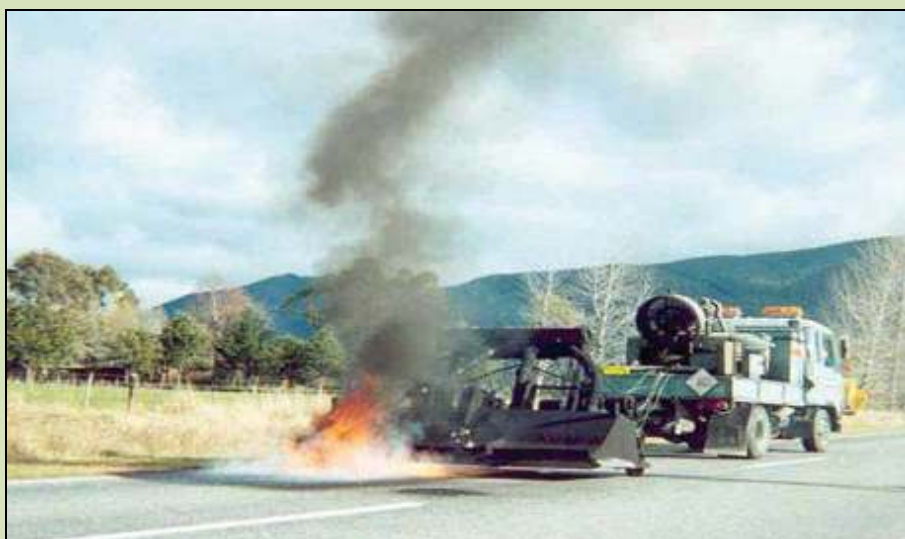
Figure 4 Burning excess bitumen from a flushed chipseal Source: Pidwerbesky, Beuzenberg & De Bono (2009) 93
