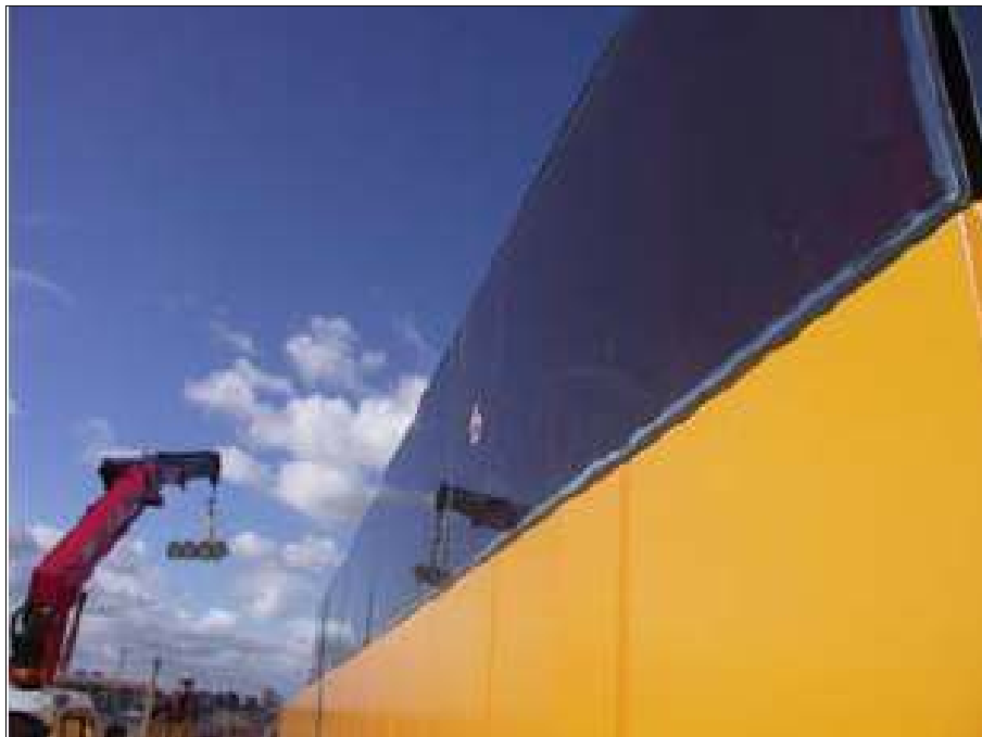
Figure 11 Solar panels on noise walls
